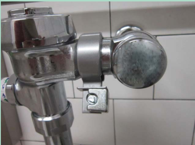
P-LOCK shown here with its' tamper resistant lock.
